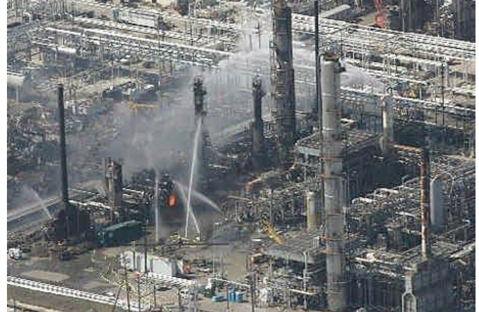
Figure 1. Damaged refinery equipment
