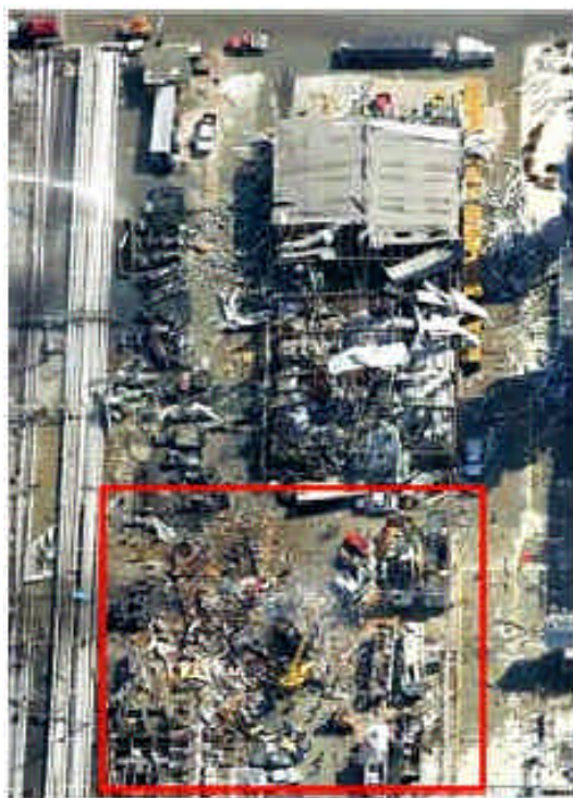
Figure 2. Aerial view showing some of the destroyed temporary trailers (inside red box)
