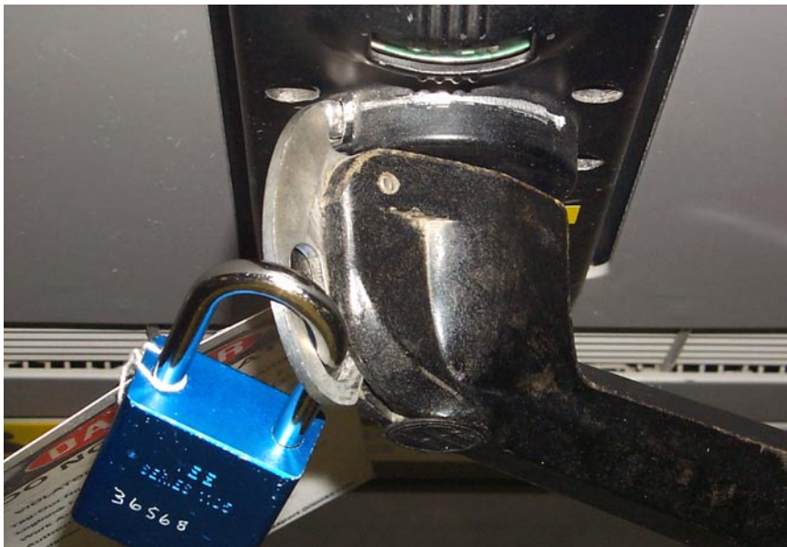
Figure 2-2. Lock installed in circuit breaker handle locking device
