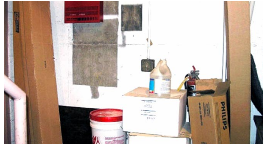
Figure 3-1. Can you find the fire extinguisher?
