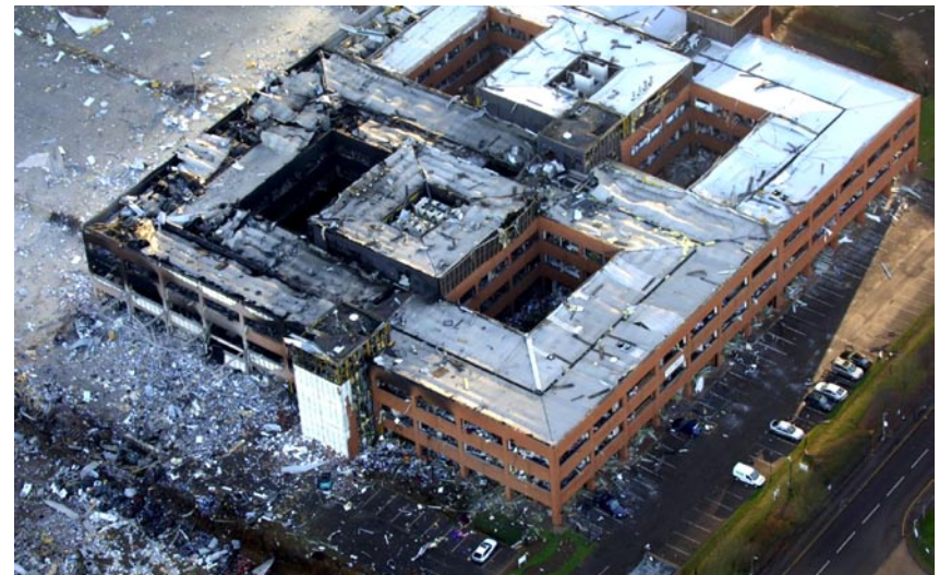
Figure 3-3. Damage to an adjacent building
