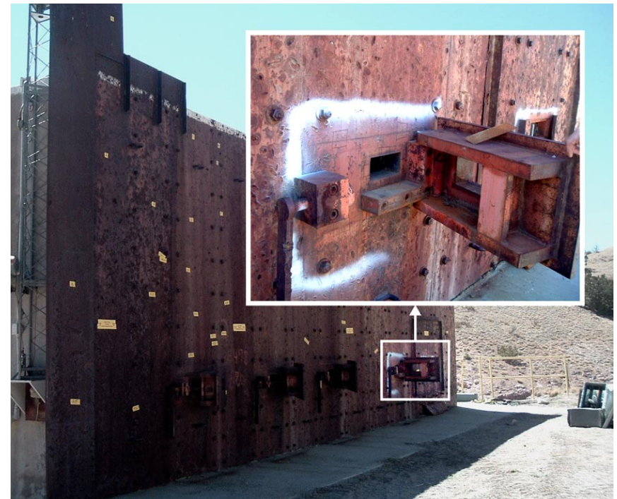
Figure 2-1. Exterior wall of building
