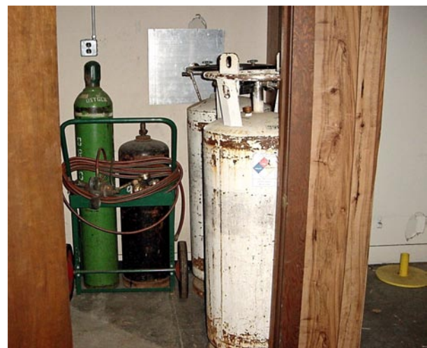
Figure 3-5. Adjoining room in basement storing combustible pressurized cylinders
