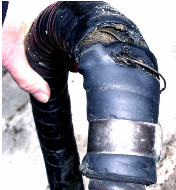
Figure 1-2. Damaged hose at nozzle connection
