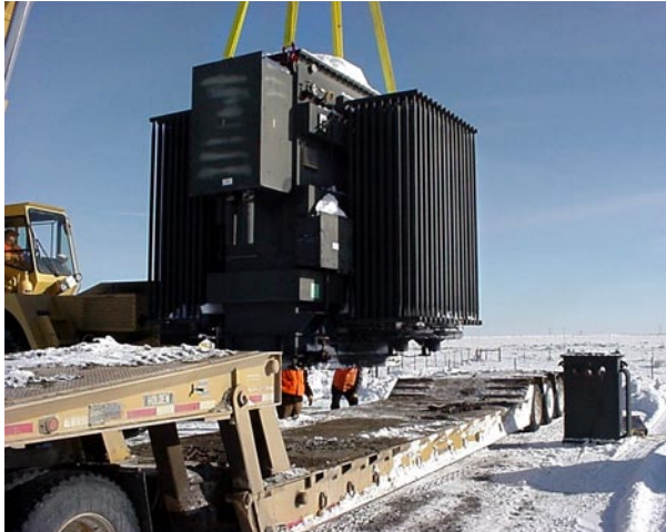
Figure 2-1. Transformer being loaded onto trailer
