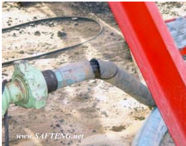
Figure 1-3. Failed return hose
