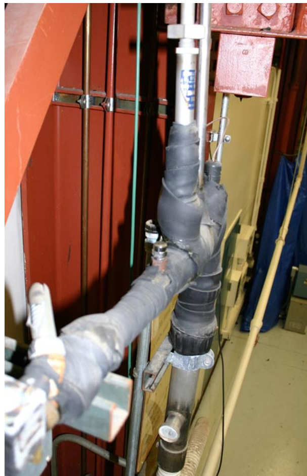
Figure 3-1. Pressure relief valve
