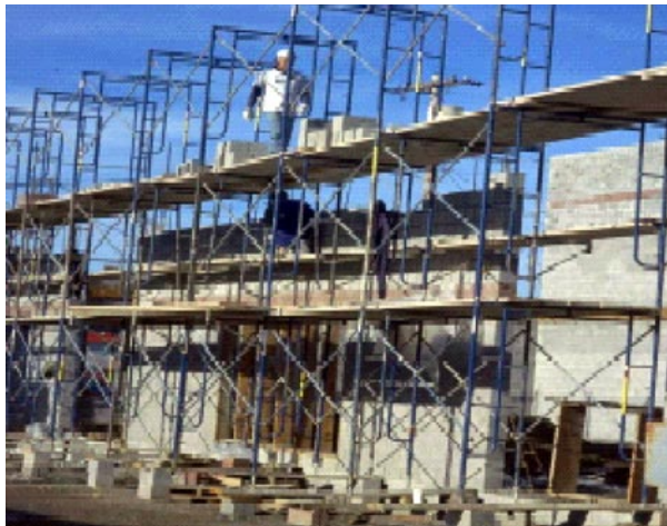
Figure 1-1. Typical worker on scaffold
