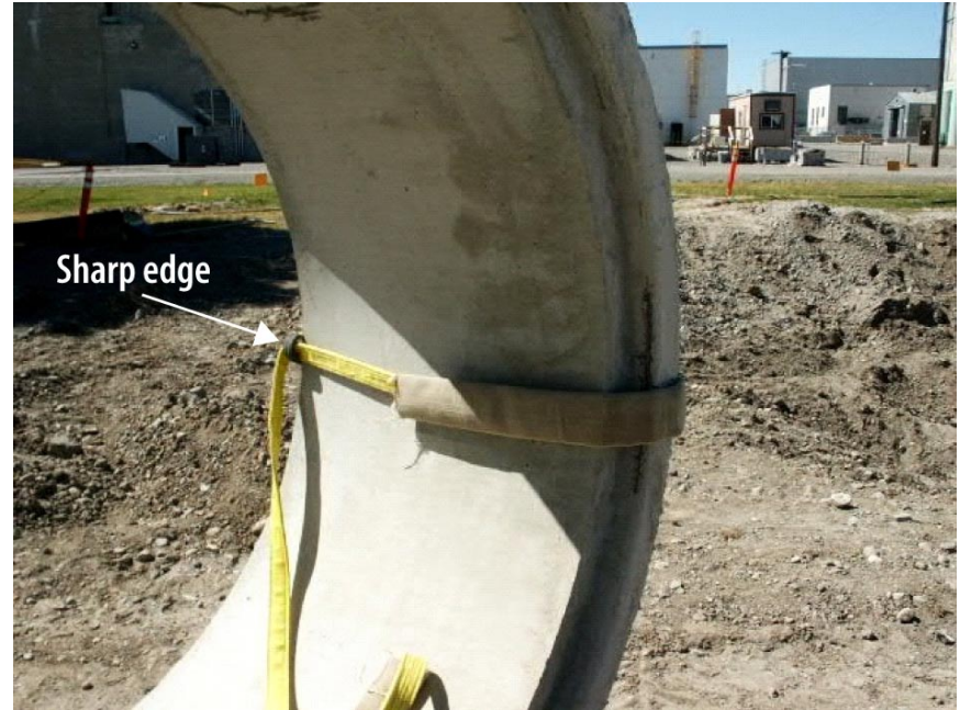
Figure 1-2. Lifting sling configuration
