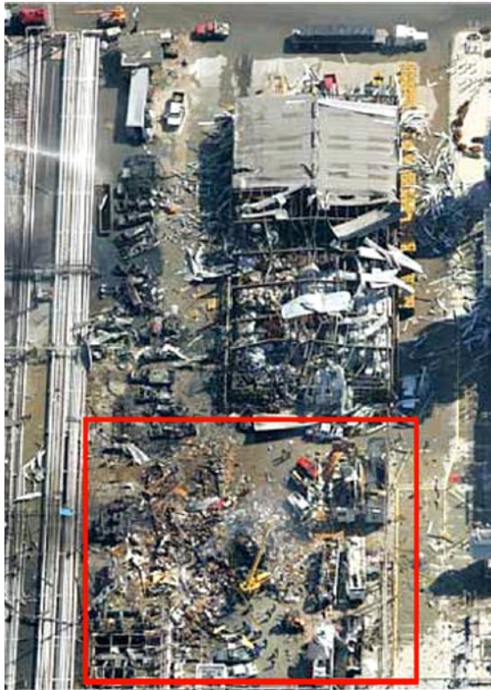
Figure 3-2. Destroyed temporary trailers (red box)
