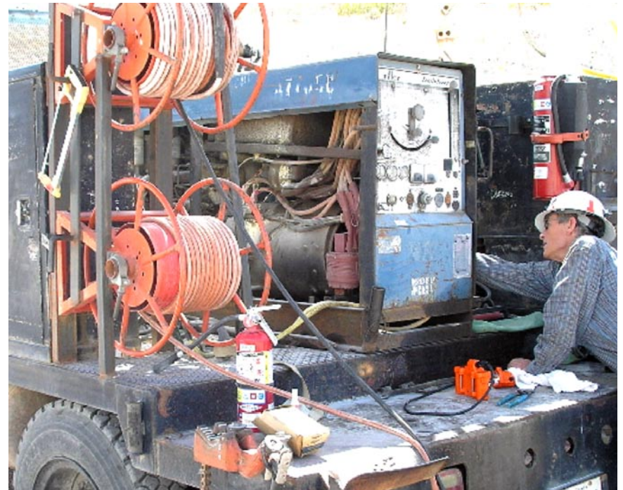
Figure 2-1. Welder/generator (blue) on bed of mechanic truck
