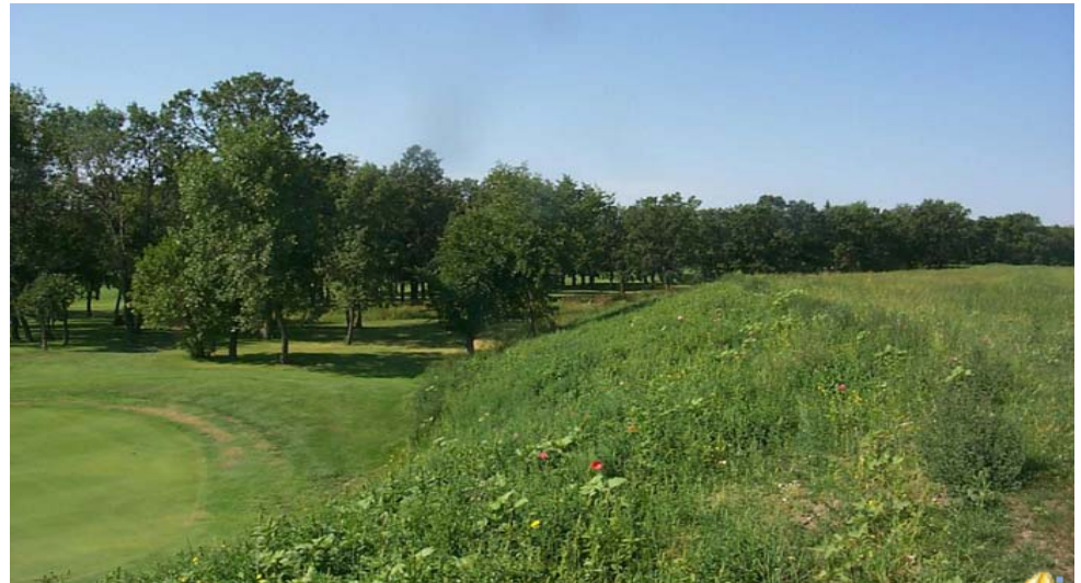
Embankment at Golf Course
