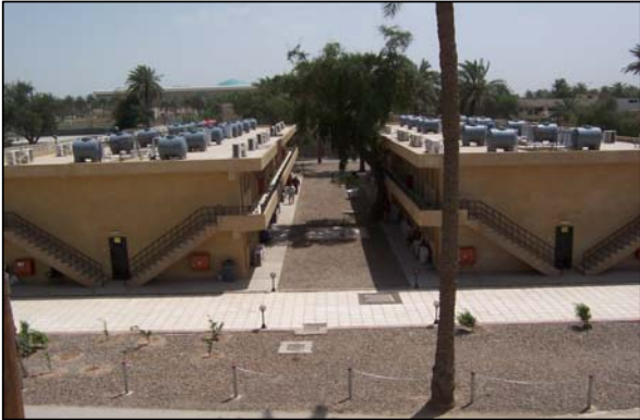
GRD HQ Billeting Additional Housing Units
