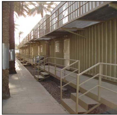
Additional GRD HQ Billeting Exterior View
