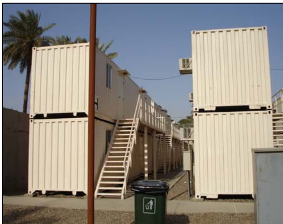
Additional GRD HQ Billeting Exterior View
