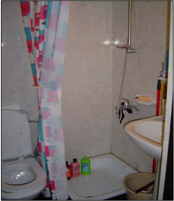
GRD HQ Billeting Bathroom
