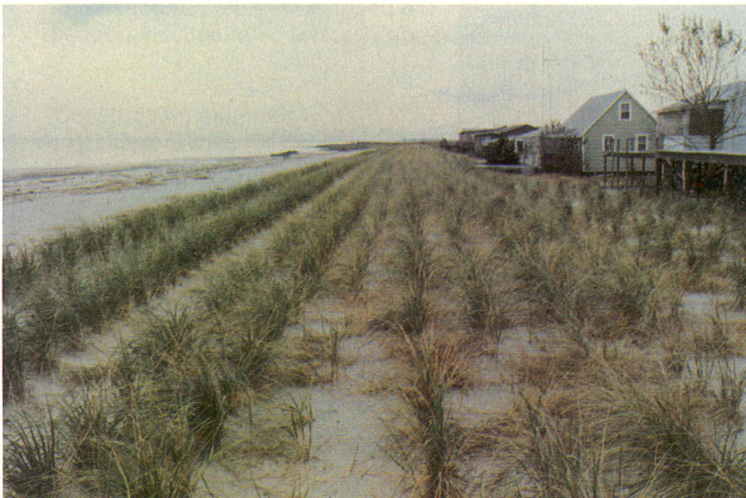
Vegetation planted for erosion control
