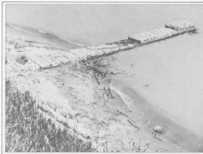
Gabion groin, 3 miles south of Port Sanilac, MI.
