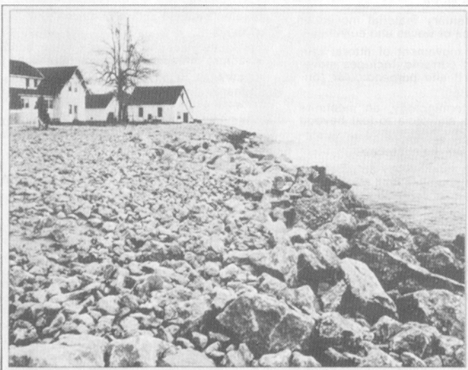
Rock revetment at Tawas Pt. MI.
