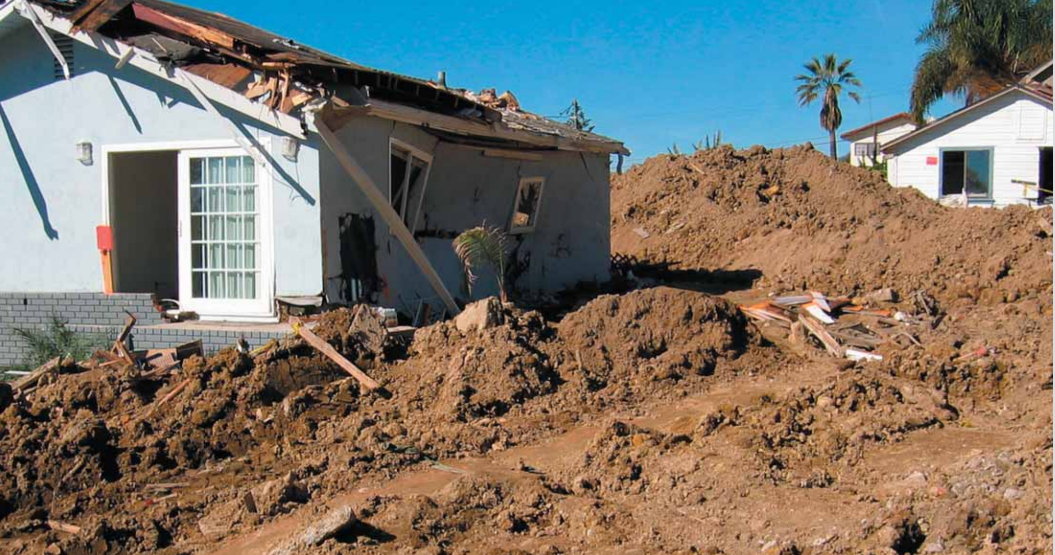
Mudslide Credit: News Photo/UNEP/FEMA
