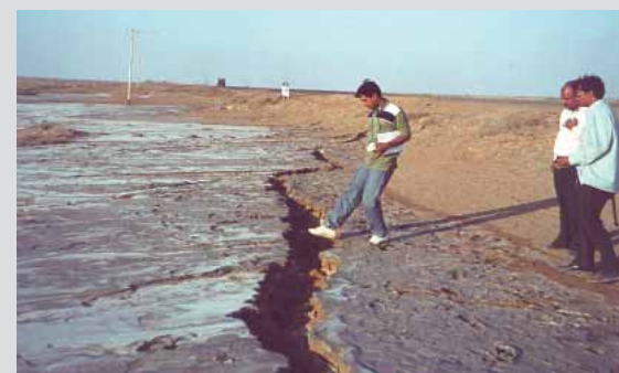
A big tentional crack (approximately 30 cm deep) in a nearby field on Bhuj, Khewda. Salt water had come up to the surface through the crack due to liquefaction. Credit: Ramesh P. Singh/UNEP/Indian Institute of Technology, Kanpur
