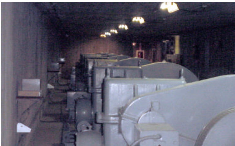
What a dam tender sees in the dungeon-like Hoist Room.
