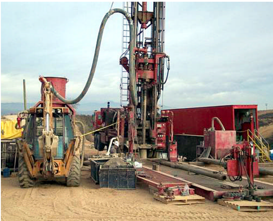
Contact crews drill wells to test groundwater.
