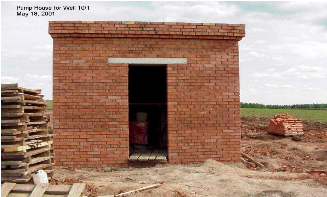
Figure C-3. One of the well houses during construction
