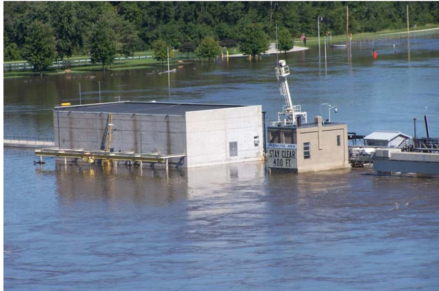
Starved Rock Lock and Dam on the Illinois River experiences record flooding in this photo taken the morning of Sept. 18. Photo by Bob Petruney, Illinois Waterway Visitor Center.
