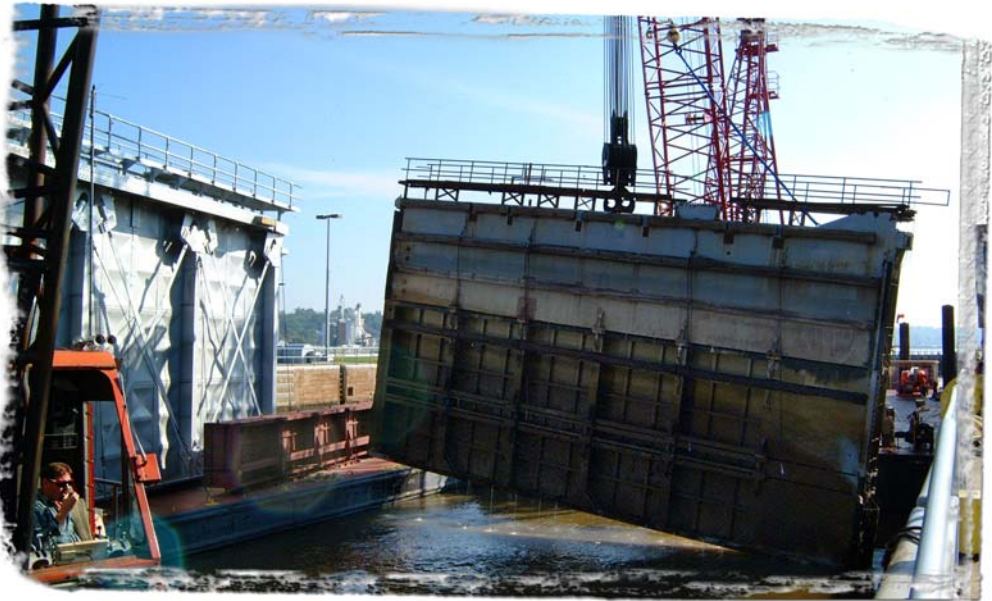
Above - Crane operator Joe Goin, Mississippi River Maintenance Crew, looks on as one of the Corps' largest cranes, the Quad-Cities, removes the first spare miter-gate and slowly moves it toward a barge where it was secured next to the renovated gates that would replace the spares.
