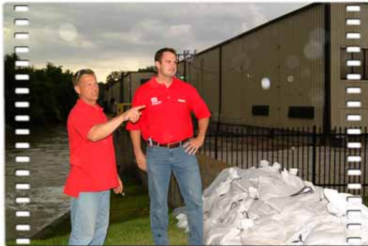
Matt Stewart listens to Randy Kinney, a geotech member of the Quincy EOC, as they both assess the effectiveness of the flood-fighting methods used in the south Quincy, Ill., area near Lock and Dam 21.
