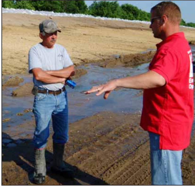
Randy Kinney, Engineering and Construction, shares his geological assessment about the seepage found at the base of the levee with a community levee inspector at the upper Indian Grave levee district near Ursa, Ill.
