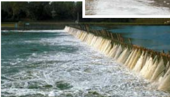
Wicket gates are hooked and stabilized to make a wicket dam on the Illinois River.
