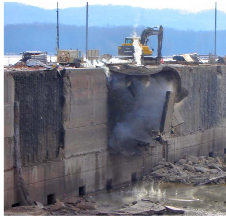
(Top photo) Ongoing work inside the lock chamber two days after blasting and cleaning debris had taken place. (Right) One of 37 blasts to remove aged vertical wall concrete inside the lock chamber. The 9 days of blasting finished with zero accidents or incidents. (Center) Contractors encase the lock's downstream bubbler pipe in concrete, while Jake Cawiezell, Engineering and Construction, oversees the progress. Photos by Jodi Bausman, Engineering and Construction.
