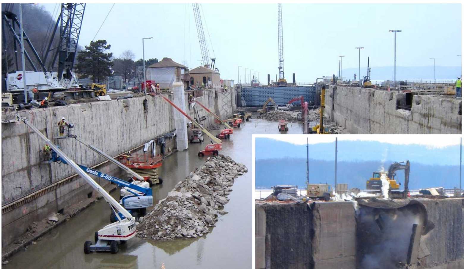
(Top photo) Ongoing work inside the lock chamber two days after blasting and cleaning debris had taken place. (Right) One of 37 blasts to remove aged vertical wall concrete inside the lock chamber. The 9 days of blasting finished with zero accidents or incidents. (Center) Contractors encase the lock's downstream bubbler pipe in concrete, while Jake Cawiezell, Engineering and Construction, oversees the progress. Photos by Jodi Bausman, Engineering and Construction.
