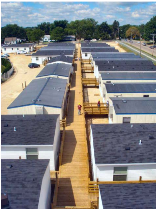
Workers can be seen on the wood decking, which connects the Cedar Rapids Community School District buildings on the grounds of Kingston Stadium. Photo courtesy of Alliant Energy.
