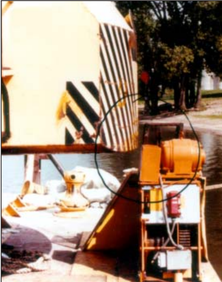
The area Lowell Sweatt's fatality occurred on Aug. 26, 1986.
