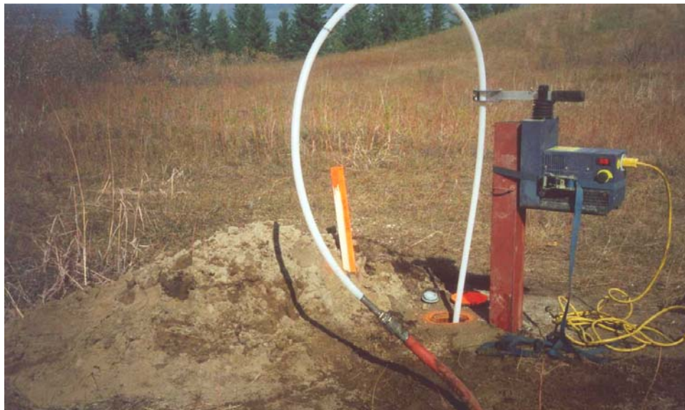
Figure 3-20. Development of wells using mechanical Waterra pump
