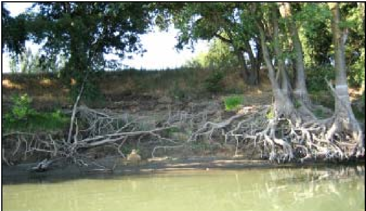
b) Site RM 48.2R waterside, July 2006, Ayres Associates.
