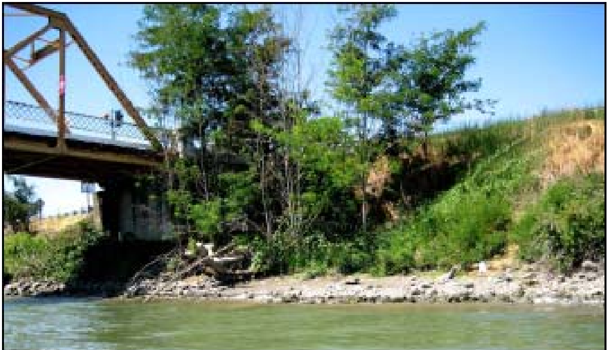
b) Site RM 33.3R waterside, July 2006, Ayres Associates.
