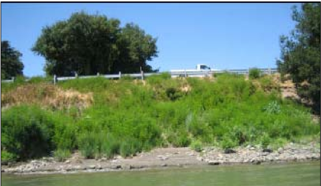
b) Site RM 33.0R waterside, July 2006, Ayres Associates.
