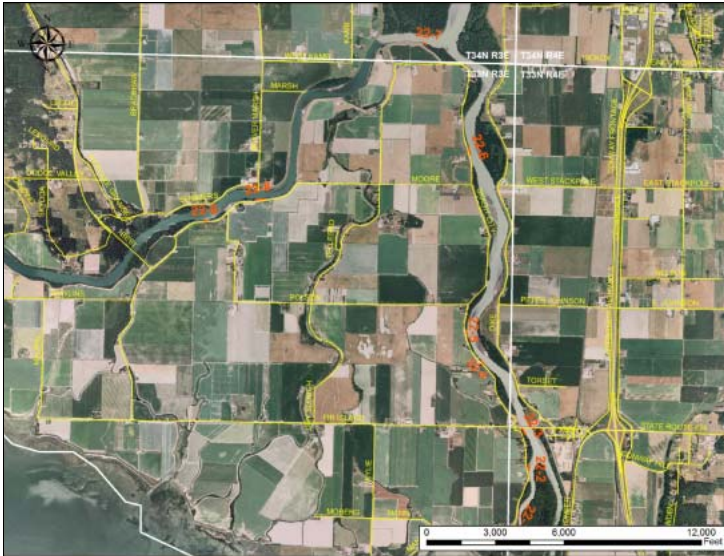
Diking District 22, Skagit County, Levee Repair Locations – 9 sites
