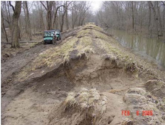
Figure 6.2 and 6.3, Levee breaches along the Wabash River
