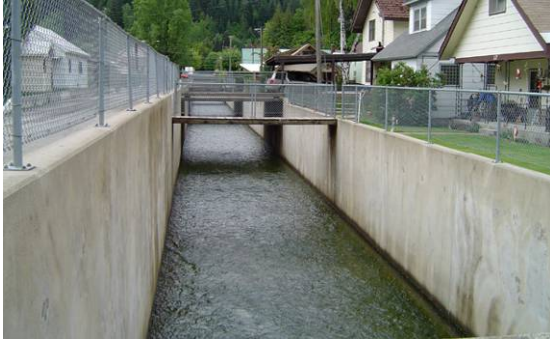
Figure 2.72 ACCEPTABLE concrete lined flood control channel. (ID)
