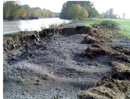
Figure 2.2 Flood damage. (WA)
