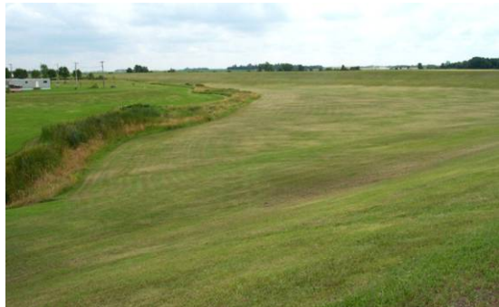
Figure 2.57 ACCEPTABLE interior ponding area and drainage ditch. (MN)
