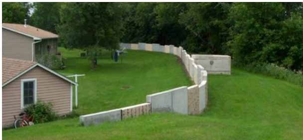
Figure 2.48 MINIMALLY ACCEPTABLE floodwall. Monolith joint separation caused by settlement, no landward or riverward tilting. The opening is about 3 inches wide at the top but the rubber joint sealer is still intact and undamaged. This joint has since been repaired by bolting another joint sealer on the both sides of the wall and filling the void with an expandable joint sealer. (ND)
