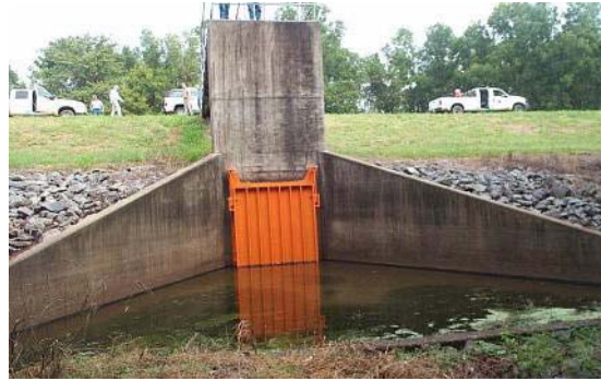
Figure 2.63 ACCEPTABLE culvert gate. (LA)
