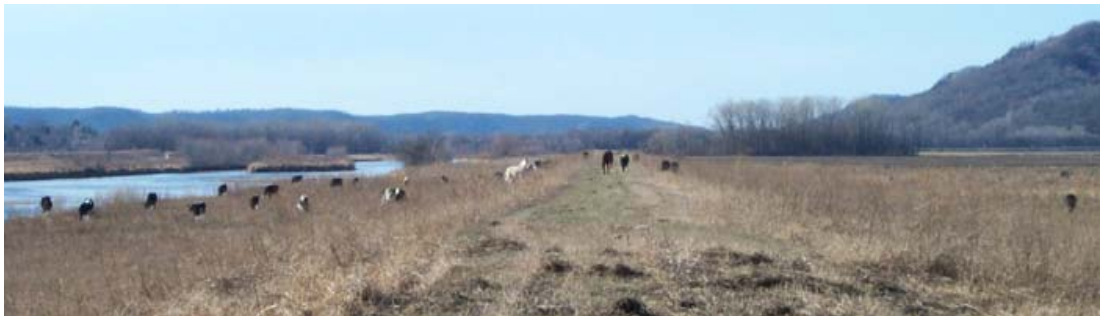
Figure 2.29 MINIMALLY ACCEPTABLE. This photo shows cattle grazing on the levee. Cattle typically don't harm the sod cover to the extent that sheep or other animals do. In this case, the landowner and the public sponsor were informed of the Corps' policy that grazing is not permitted on levees or within the levee easement area.
