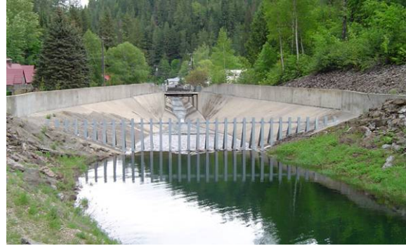
Figure 2.73 ACCEPTABLE intake structure upstream of the concrete channel. (ID)
