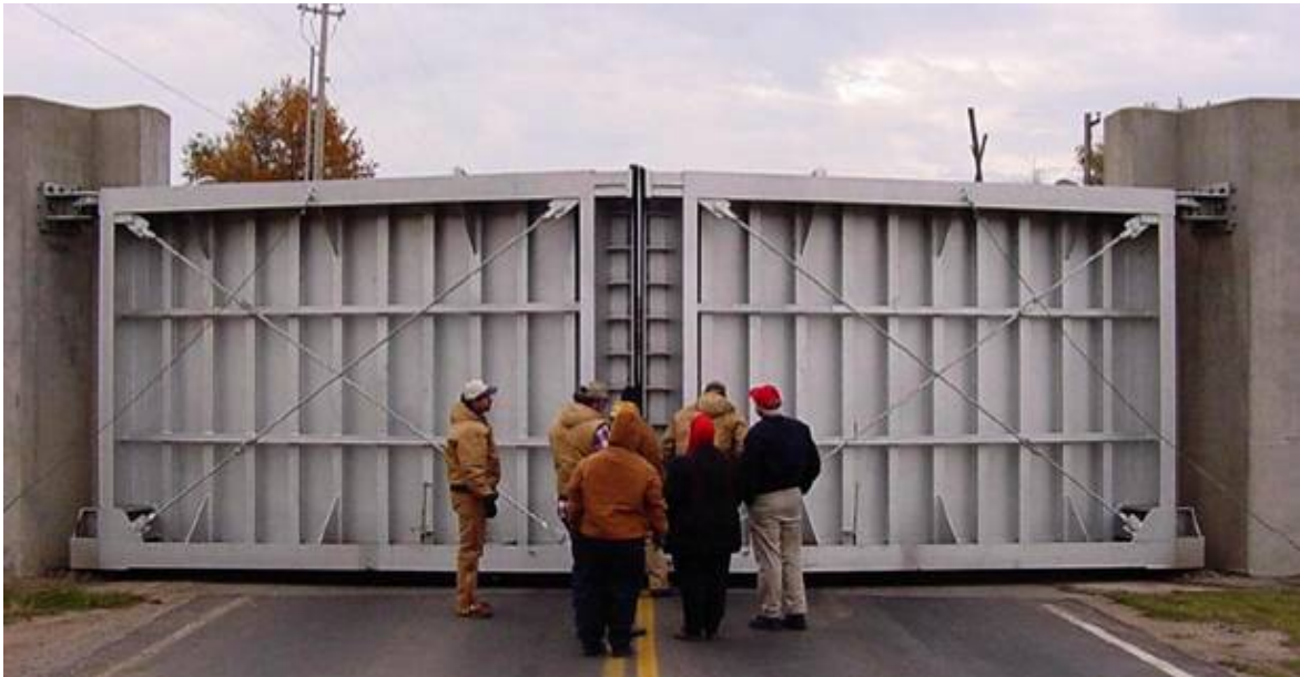
Figure 2.42 ACCEPTABLE floodgate in a levee. (KS)
