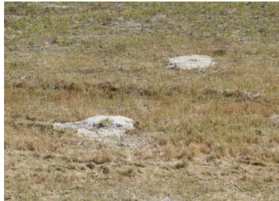
Figure 2.41 Evidence of sandboils. (IN)
