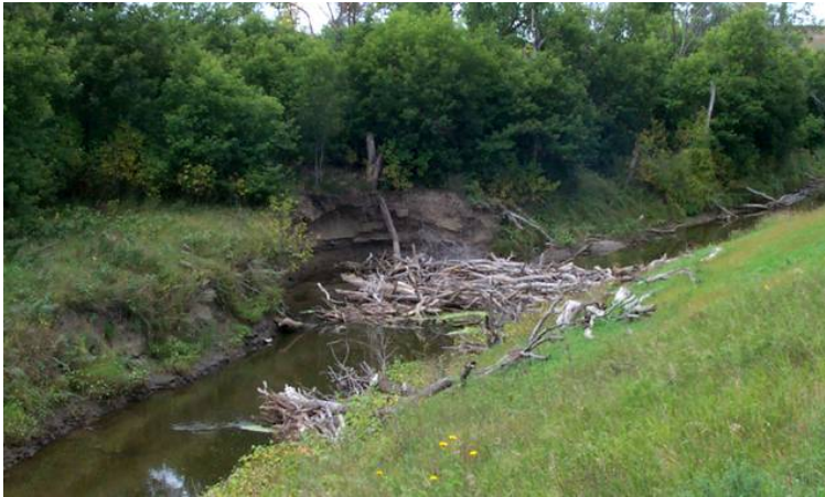
Figure 2.19 UNACCEPTABLE erosion of river channel, caused by a log jam. (ND)
