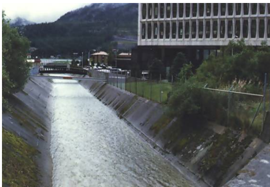
Figure 2.74 ACCEPTABLE concrete lined channel. (AK)
