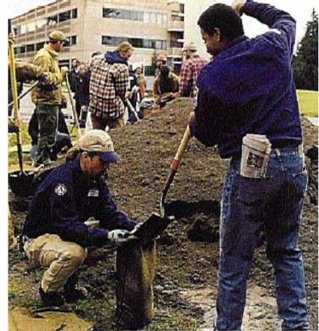
Figure D.1 This two-person team is positioned properly for sandbag filling.
