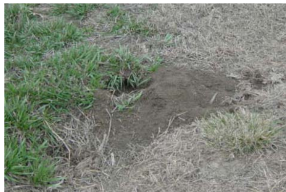
Figure 2.20 Animal burrow in a levee. (IA)
