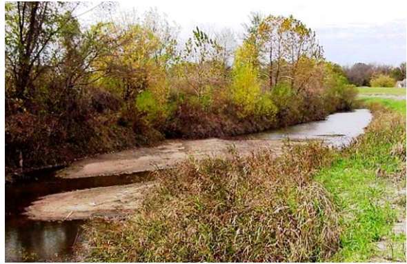
Figure 2.69 UNACCEPTABLE vegetation in channel and sediment shoaling. (OK)
