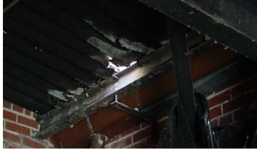
Figure 2.67 Hole in roof of pumping station. (IL)
