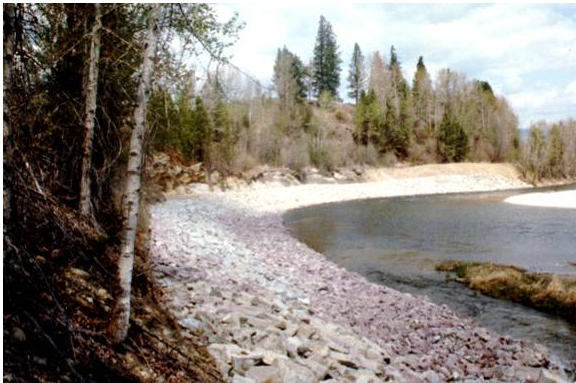
Figure 2.25 ACCEPTABLE riprap for erosion control. (MT)
