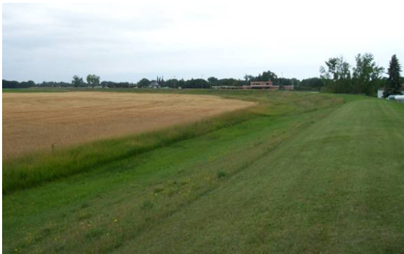
Figure 2.4 ACCEPTABLE. Landowner has not encroached on levee easement area and has stayed back 10 - 15 feet. (MN)
