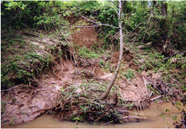
Figure 2.18 Classic picture of a tree causing slope failure. (WA)
