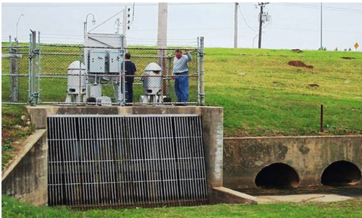
Figure 2.68 Pump station beside earthen levee. (OK)
