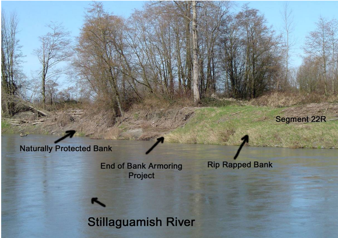
Figure 2.23 Flood damage on a naturally protected bank, as compared to damage on an adjacent bank which was protected with riprap. (Note that even though the riprap clearly protected the area during the flood, if it was observed an inspection it would have probably been rated Minimally Acceptable because the grass would have prevented an inspector from properly examining the riprap.) (WA)
