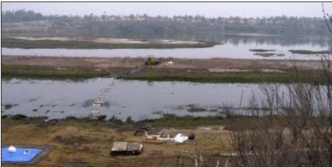
Construction Equipment and temporary bridge March 15, Hotdog Island.
