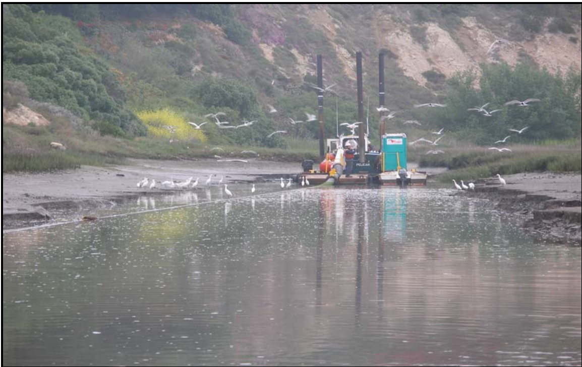
Hydraulic Dredge "Pelican" dredging Middle Island Restoration Channel, May 2006
