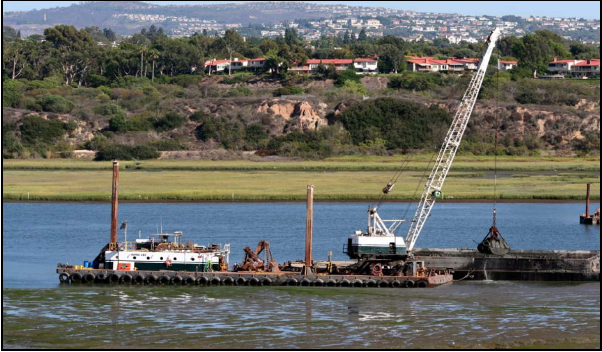
DB-3 dredging Unit II Sediment Control Basin, 29 August 2007
