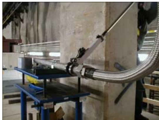
Exhibit 4-6: Ceramic Pipe Joint Repair on NuMI Horn 2.
