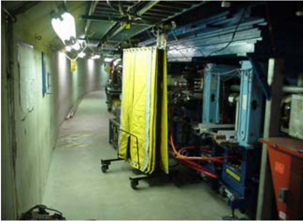
Exhibit 4-4: Shield Wall Used During Installation of Piping Manifolds in Booster Tunnel.
