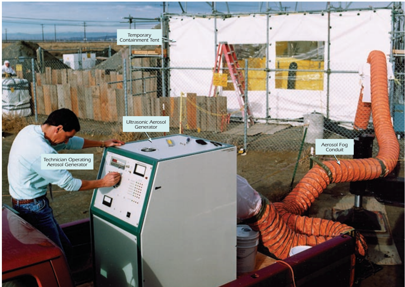
Exhibit 4-2: Aerosol Generator Used to Reduce the Spread of Contamination at Hanford
