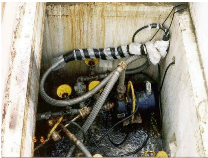
Exhibit 4-3: Contaminated Pit at the Hanford Tank Farm.
