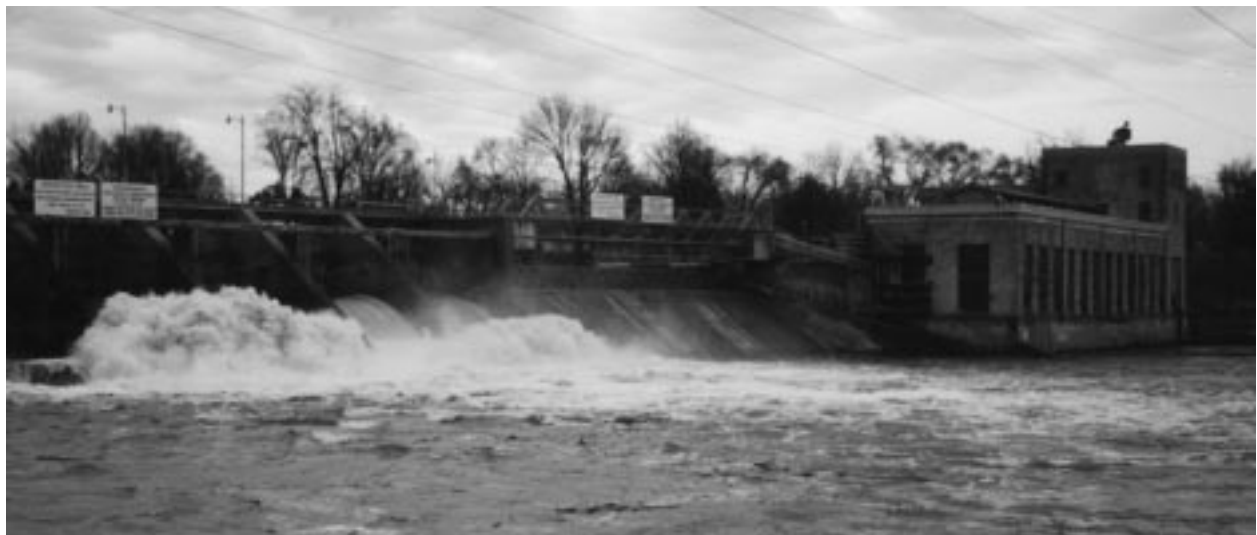
Figure 4. Example of a developed hydroelectric plant in Indiana. This Hydroelectric plant and dam is the Twin Branch plant, on the St. Joseph River, with 4.8 megawatts of installed capacity. The additional undeveloped hydropower potential at this site is 3.8 megawatts.
