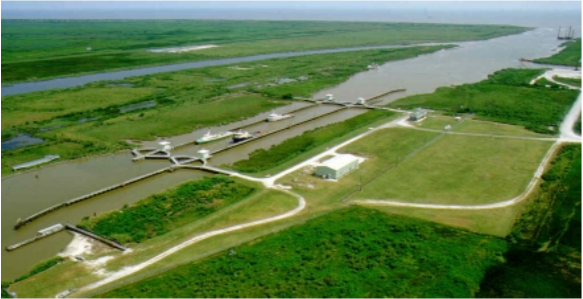
Freshwater Bayou Lock
