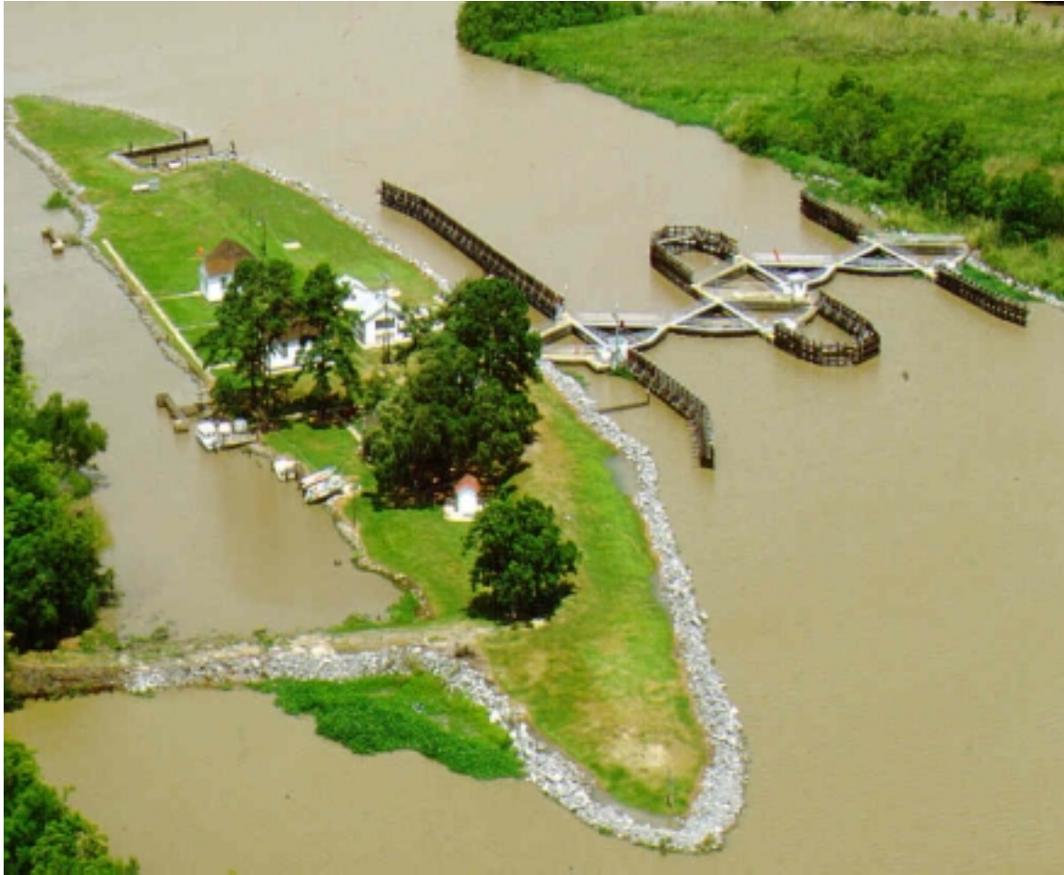
Schooner Bayou Lock
