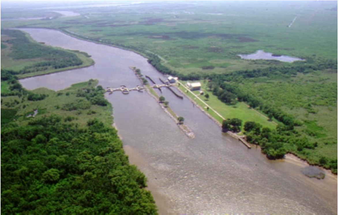
Catfish Point Control Structure
