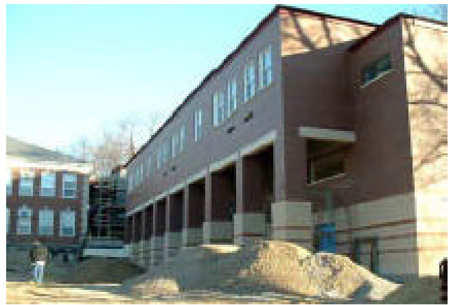
Key Elementary School construction
