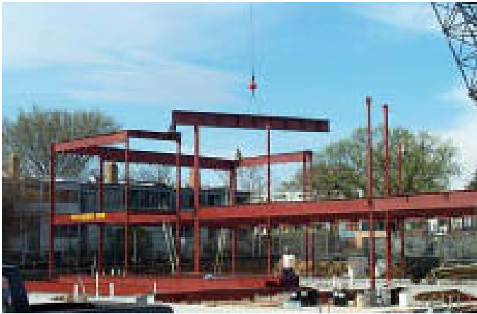
Miner Elementary School construction
