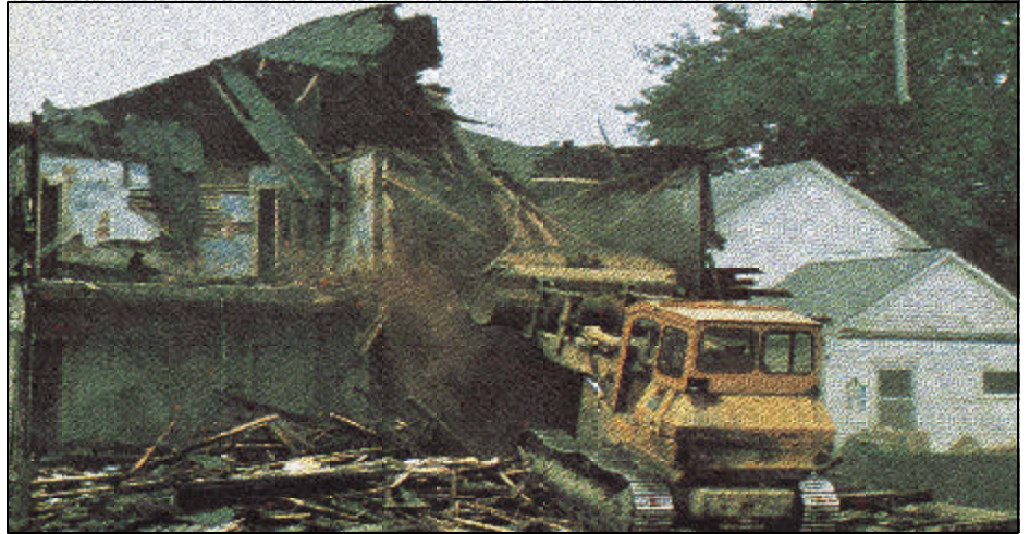
A house is demolished. The Corps bulldozed thousands of similar buildings.
