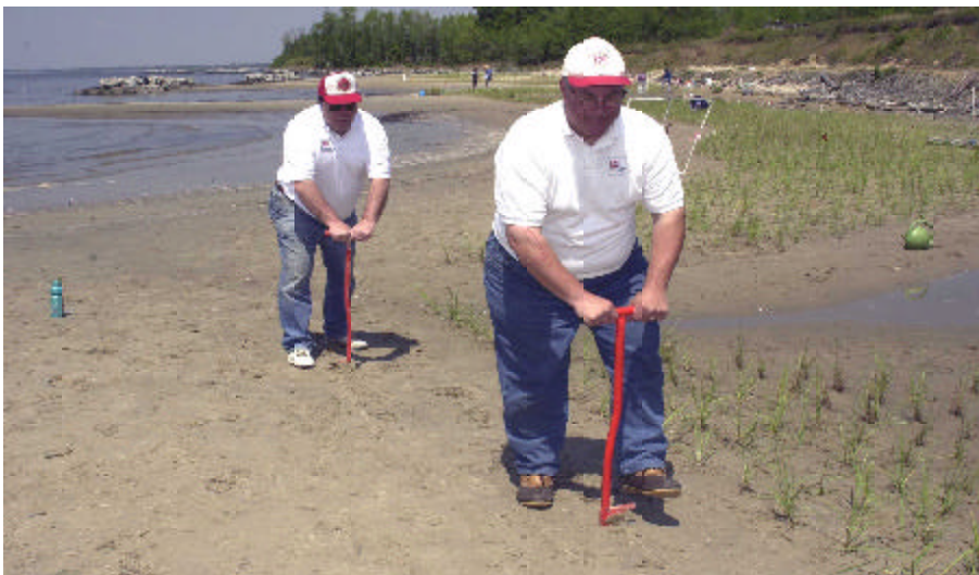
Bob Blama and Stan Snarski, Operations, demonstrate the technique of making holes approximately every 18 inches for the plants.
