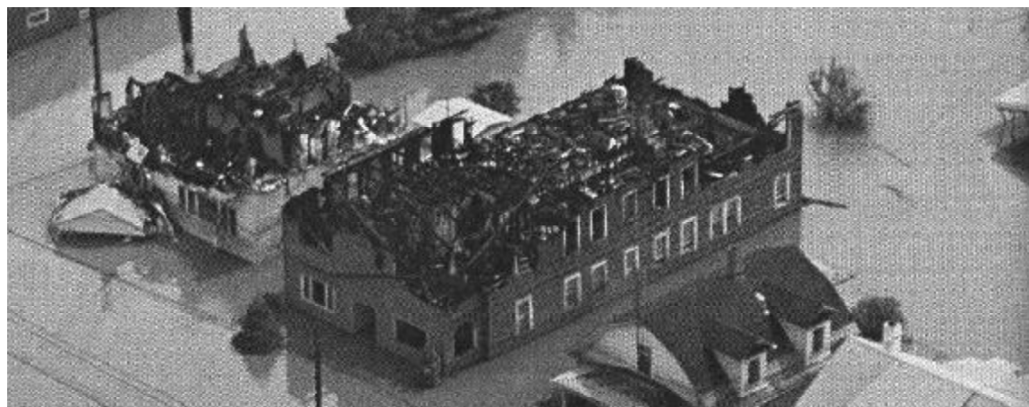
Tropical Storm Agnes left flooding and devastation throughout the Mid-Atlantic area in 1972.
