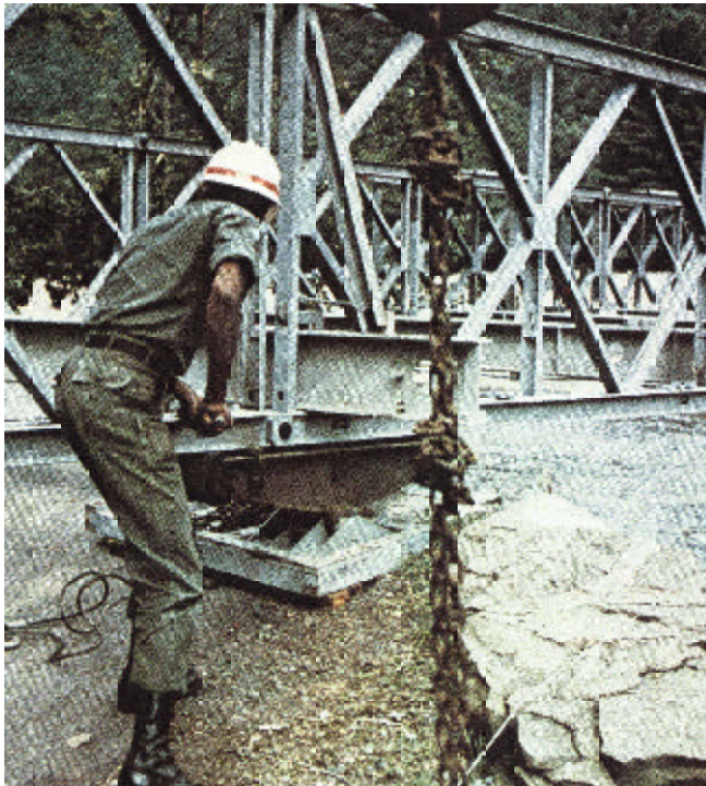
A soldier helps to install a Bailey Bridge.
