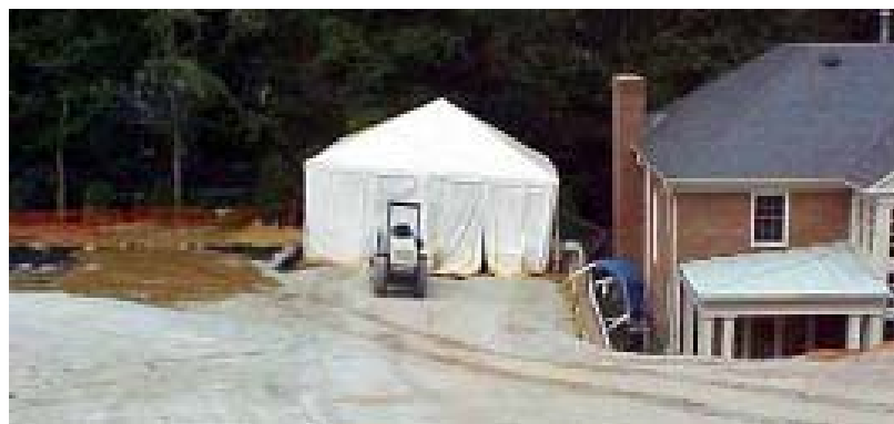
An engineering control structure, similar in appearance to this tent set up at another site, will be used at Lot 18.
