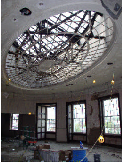
Left, the reading room in the media center during renovation. Right, work on the reading room included restoring the skylight and ceiling plasterwork, wood casing trim and two circular vestibules. New furnishings will be added.
