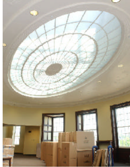
Left, the reading room in the media center during renovation. Right, work on the reading room included restoring the skylight and ceiling plasterwork, wood casing trim and two circular vestibules. New furnishings will be added.
