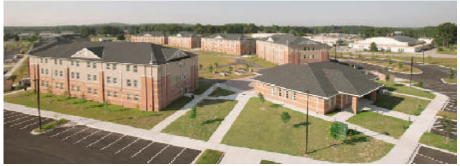
The new barracks complex at Fort Meade was completed in summer 2003.
