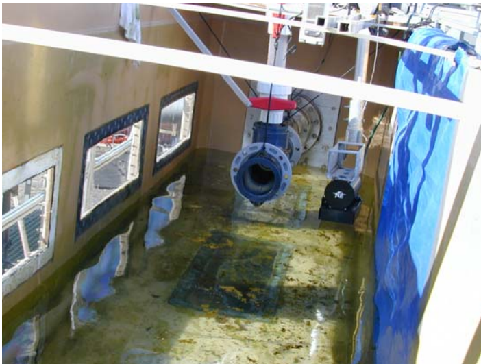
Figure 5. Induction pipe (left) and DIDSON (right) mounted in the test flume.
