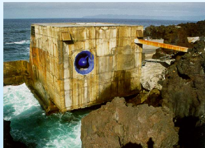
400 kW (1998), Pico Island (Azores) Fully automated, full-scale testing facility
