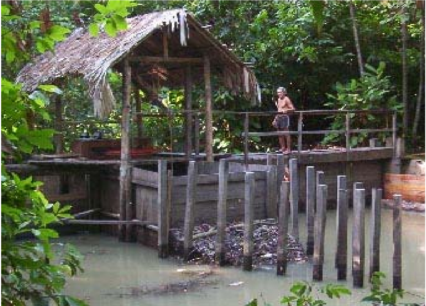
Figure 2. Field Research Station: managing tidal flow with jetties, a duct, and a gate
