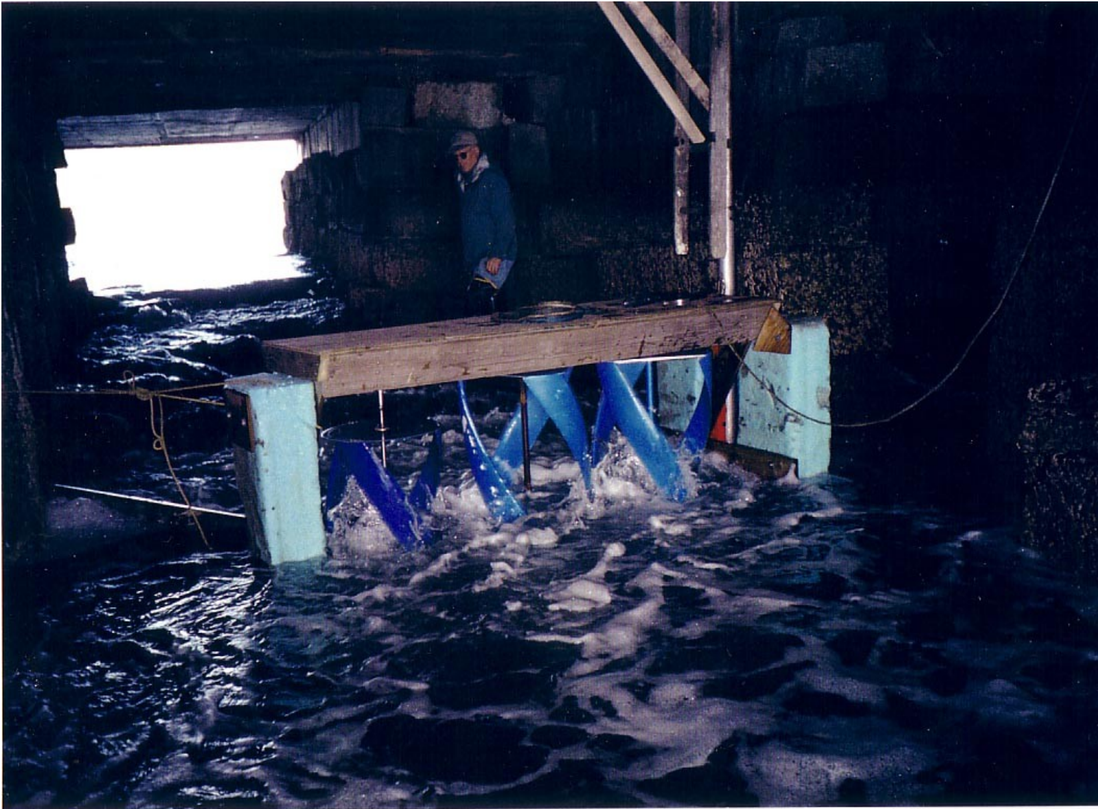
Tidal power system with three GHTs under motel, Maine, 5/03
