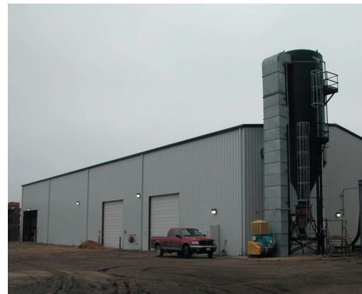
Biomass silo at Ottumwa Generating Station.
