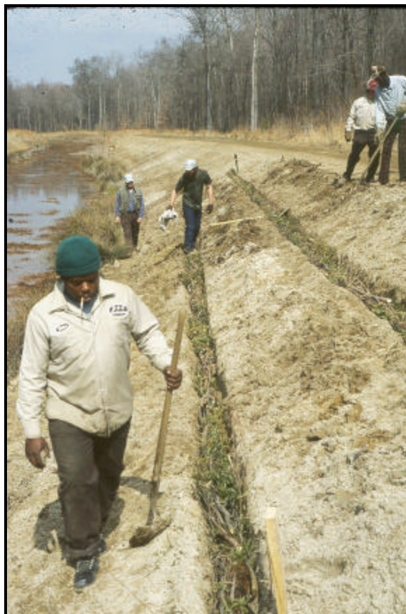
Figure 3. Installing a live fascine structure
