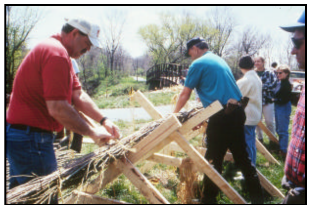
Figure 1. Building a live fascine structure
