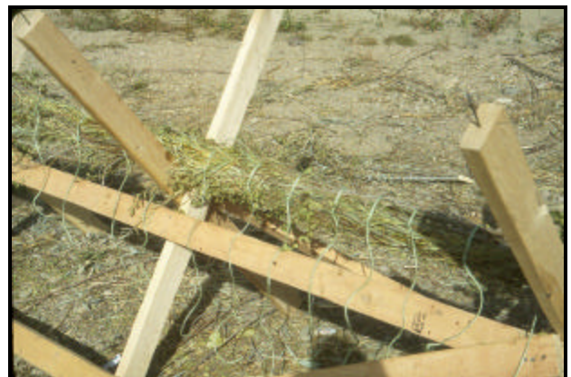
Figure 2. A fabricated live fascine structure
