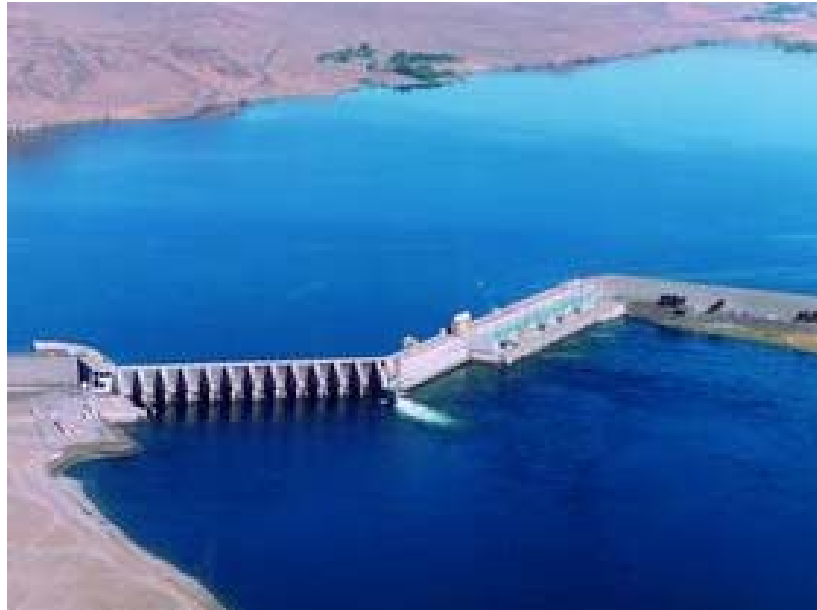
Figure 2.2. Wanapum Dam on the Columbia River, Washington. The spillway is on the left, the powerhouse is in the center, and the earth fill section is on the right.
