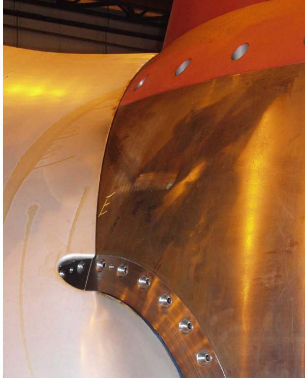
Figure 2.8. Unit 8 (AHT) Detailed View of Hub Showing the Reduced Gap between the Runner and Spherical Hub (photo provided by Voith Siemens Hydropower)
