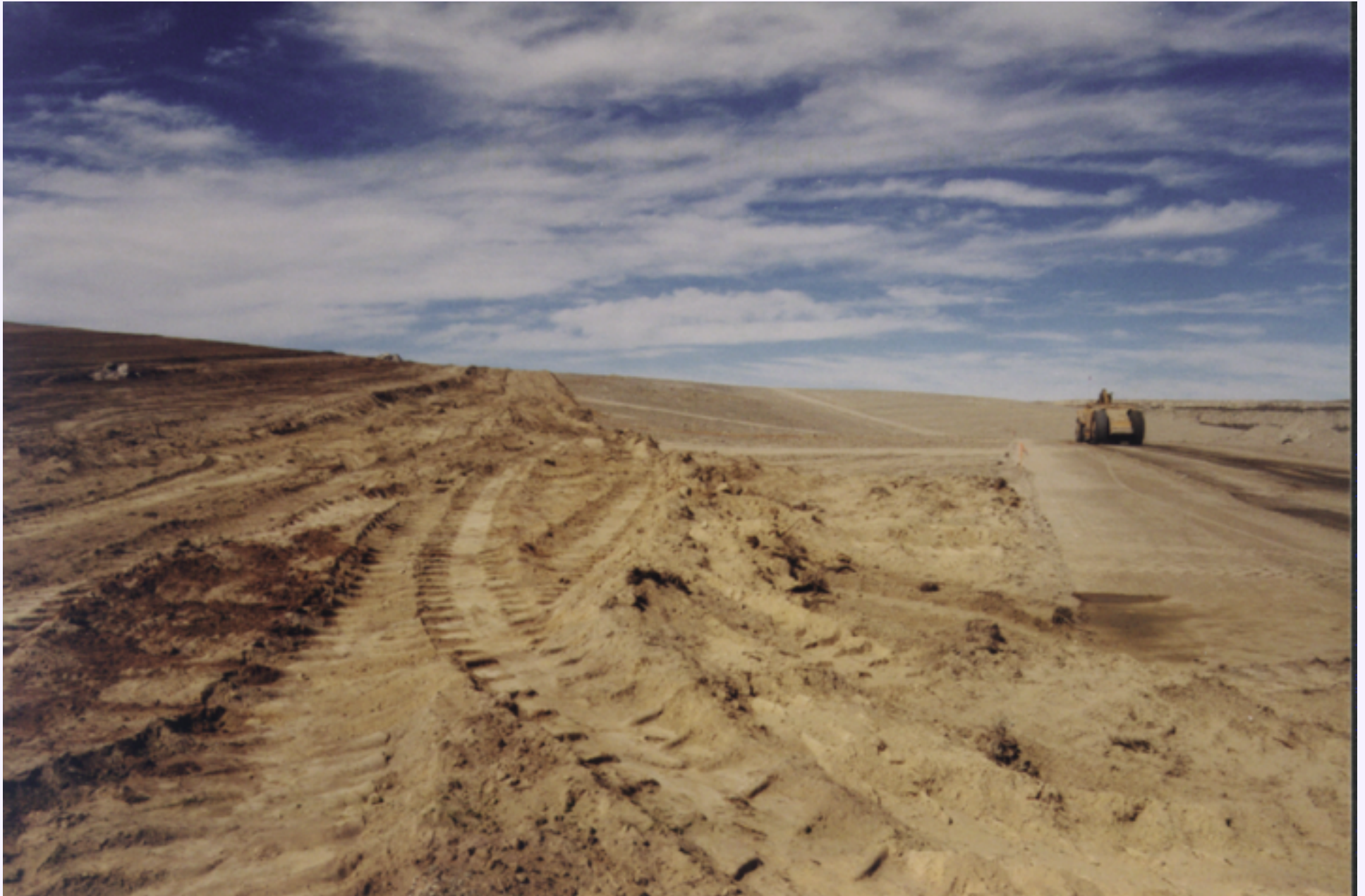
Figure MO-50. Topsoil replacement using Caterpillar scrapers.
