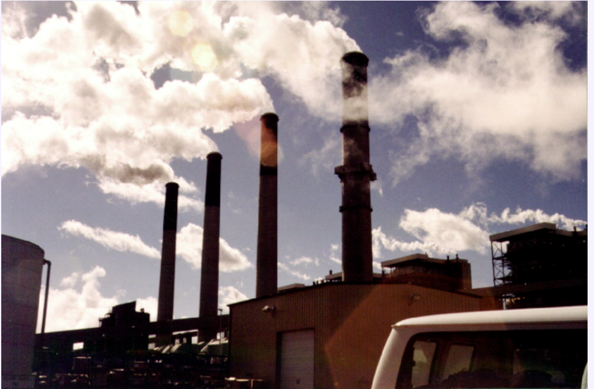
Figure MO-45. An example of a "mine mouth" power plant.
