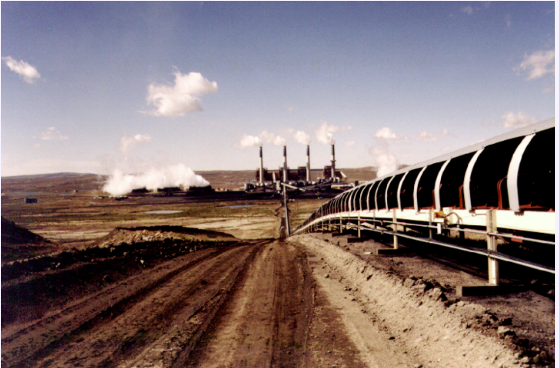
Figure MO-44. Coal is delivered to this power plant via a long overland conveyor.
