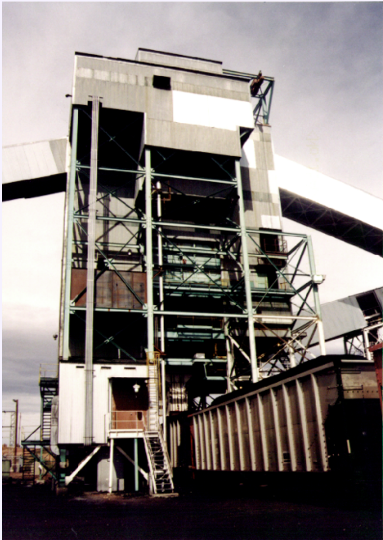
Figure MO-41. This modern train loadout provides batch loading, to fill each car to capacity, and allows different coals to be blended to meet exact quality specifications. Photograph by Ken Takahashi, 1999
