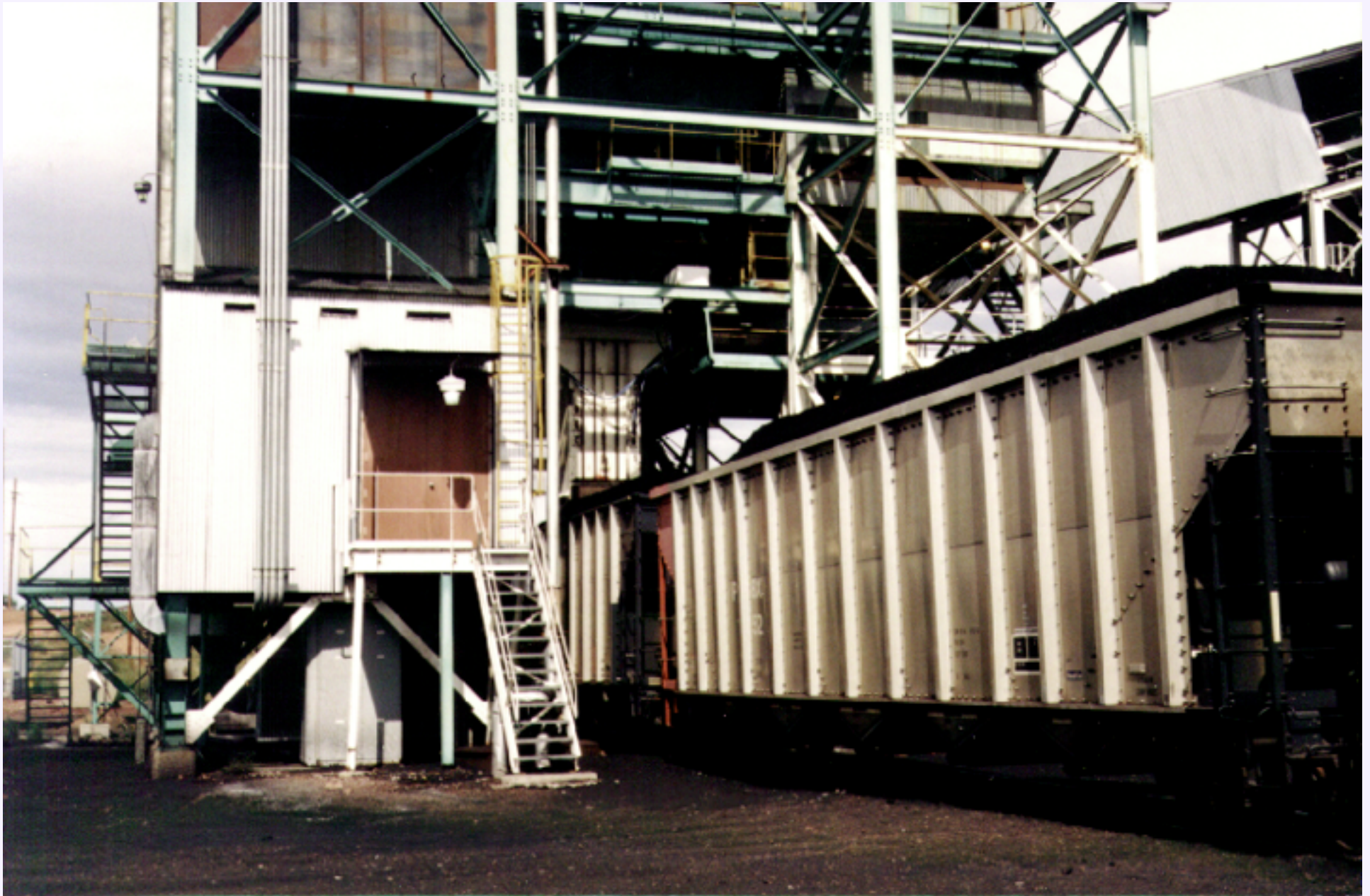
Figure MO-42. A single loadout operator with a computer system handles the coal loading and on-line sampling as the train moves forward at a speed of from 0.25 to 0.5 mile per hour. Trains must be loaded within 4 hours of arrival.
