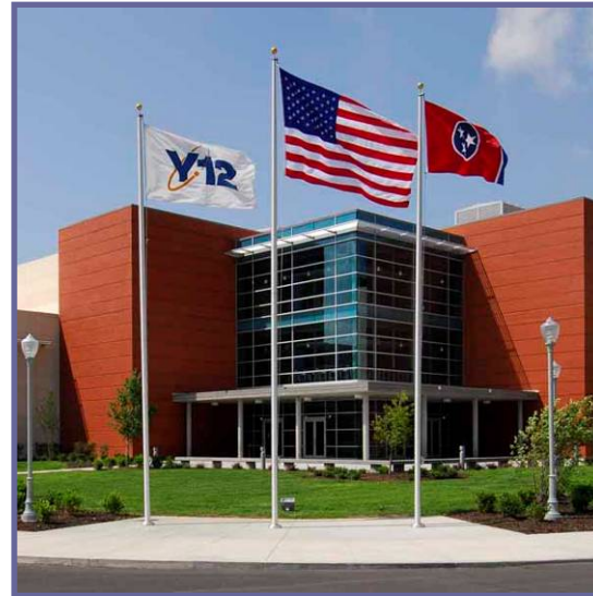
Demolition of Building 9720-6 ( upper ) and the new, alternatively financed Jack Case Center ( lower ).
