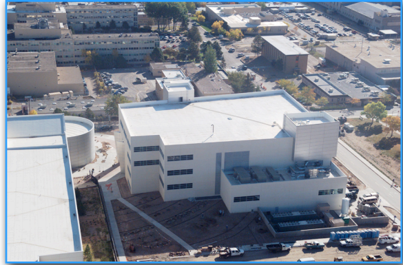
Although the NISC is a notable exception, many of the structures that support Threat Reduction are old and deteriorating.
