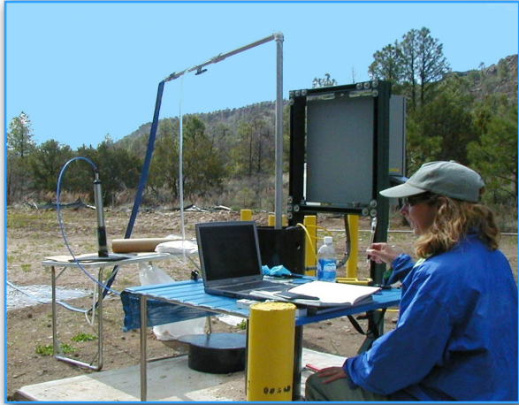
The installation of groundwater monitoring wells is included under the investigation and corrective action phases of the Consent Order.
