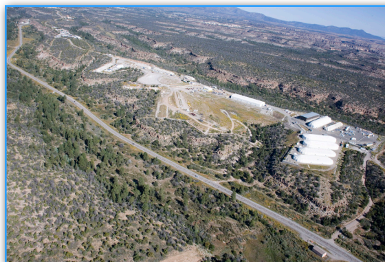
TA-54, as seen from the air, contains numerous sprung-structure domes storing TRU waste awaiting shipment to WIPP.
