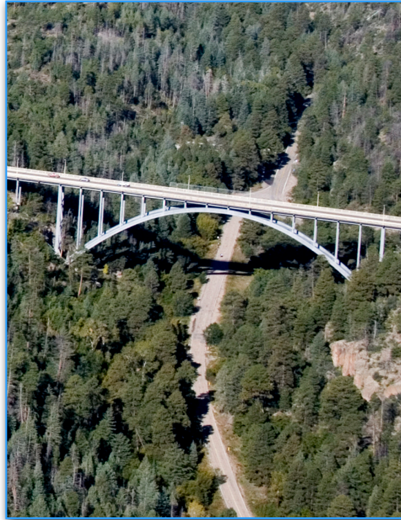
The Omega Bridge, constructed in 1951, is in need of significant maintenance within the next ten years due to deterioration of the concrete decking and seismic compliance concerns.
