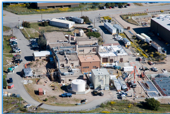
The RLWTF upgrade will enhance reliability and process capability to meet projected regulatory requirements for discharge.
