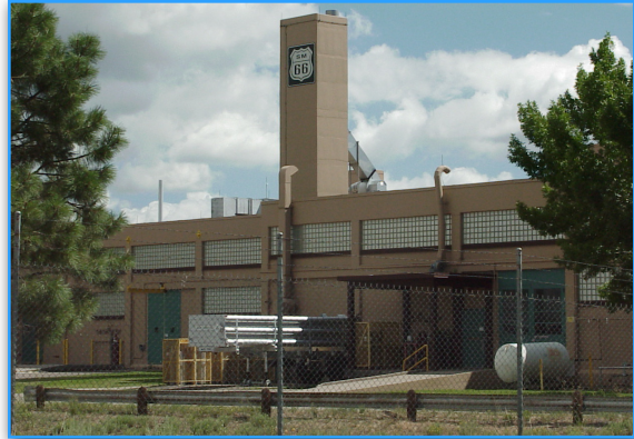
Capabilities provided by the Sigma facility will be required to support increased manufacturing under Complex Transformation.
