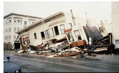
1994 Northridge Earthquake, Los Angeles (NIST)
